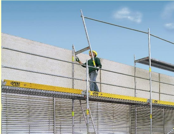
Assembly and Disassembly from the lower level – “guardrail in advance”
