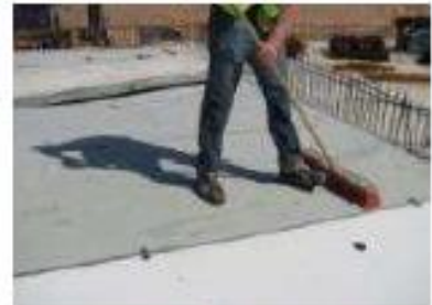
3. Remove concrete residues with a broom.
