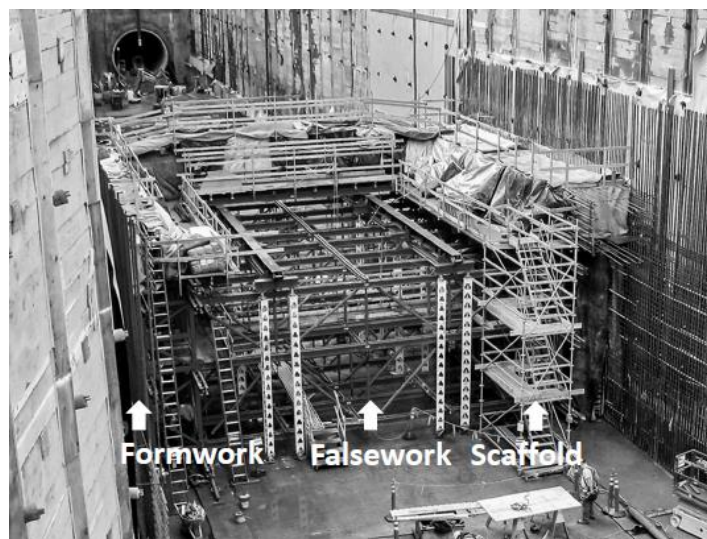
Fig. 2: Differentiation Formwork – Falsework – Scaffold [Source: C.Motzko]
