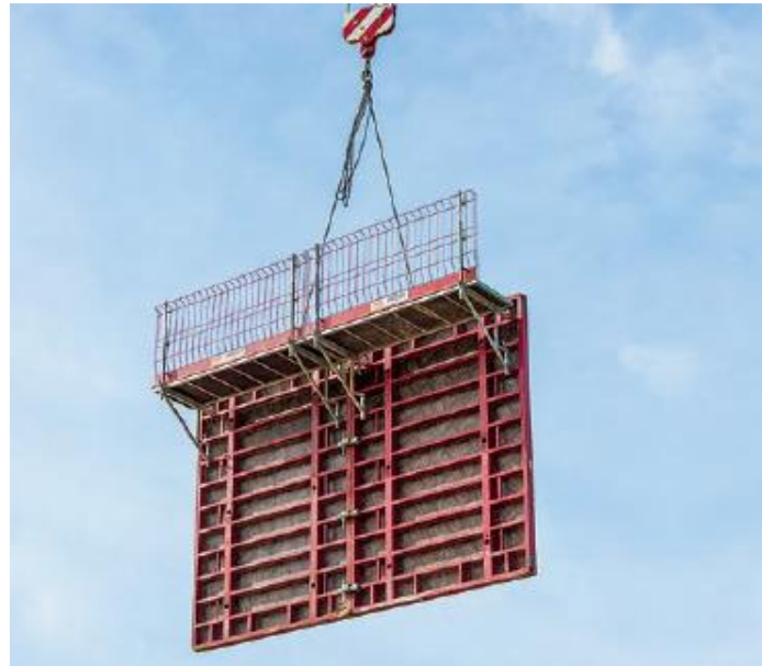
Fig. Transportation of assembled formwork fragment [Source: PERI]
