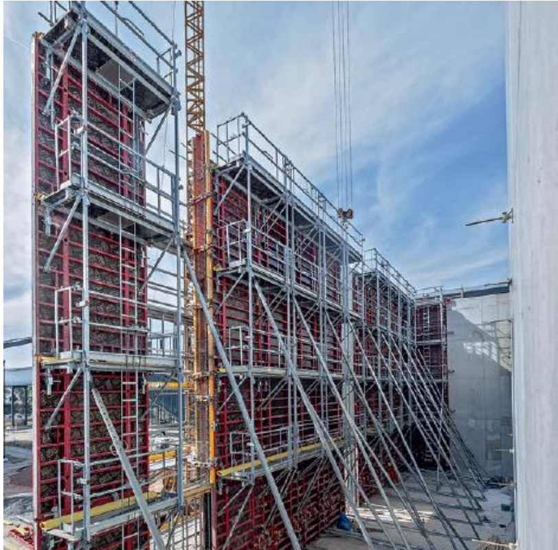
Fig. Protective handrails and assembled formwork fragment [Source: PERI]
