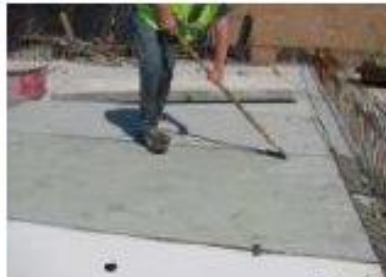
2. Remove concrete residues with a metal scraper.
